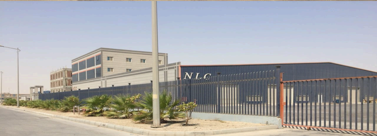
National Lighting Company Factory Location: Dammam, K.S.A
