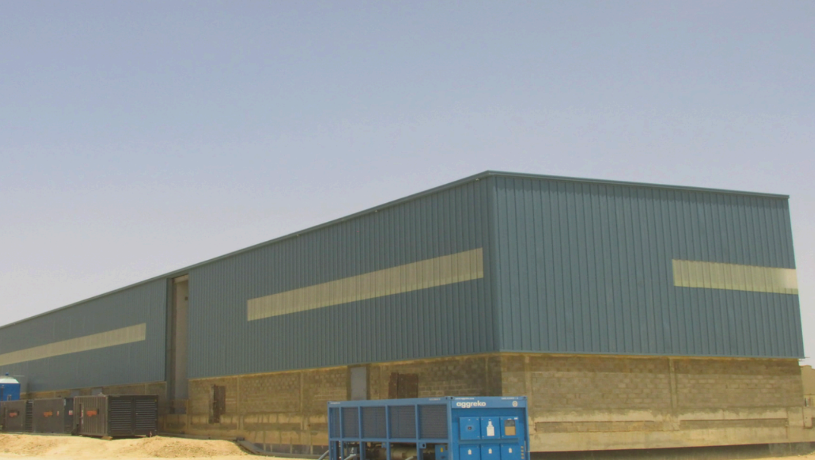
Copper Smelting Co. Plant Location: Sudair, Riyadh, K.S.A
